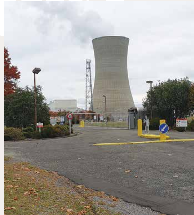
Ohaki geothermal power station
